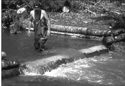
Digger Log being placed in a stream
