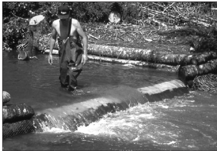
Digger Log being placed in a stream
