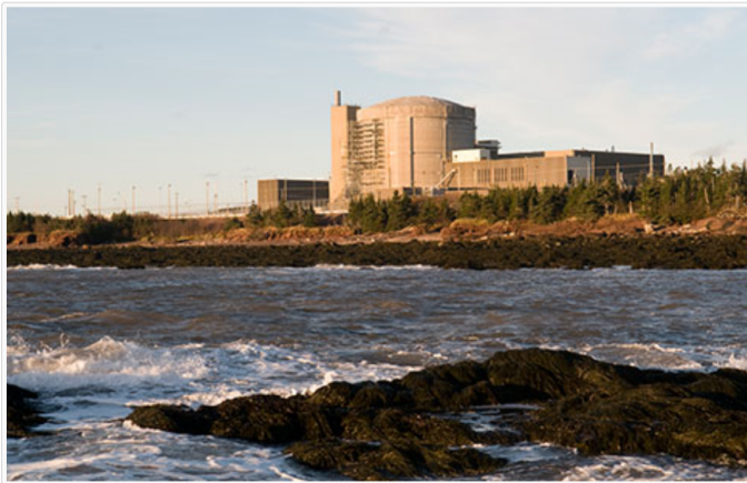
View of the Point Lepreau Generating Station
