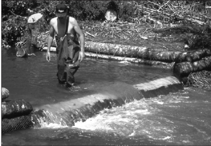
Digger Log being placed in a stream
