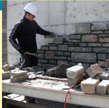
Jani Mroshaj uses a level to make sure the stone he just placed in this wall is straight.
