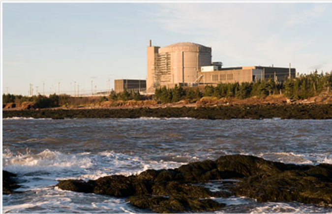
View of the Point Lepreau Generating Station
